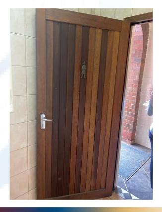
Door timber frame and door panel to be cleaned and sanded down to receive new varnish paint.
