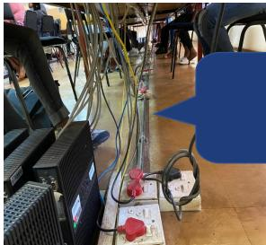
Installation of the new power skirting underneath the computer desks complete with accessories.
