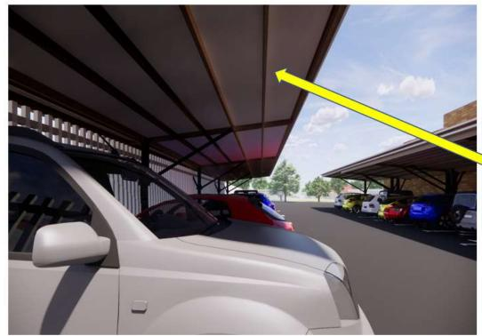
Supply and install structural steel carports as per drawings and specifications.
